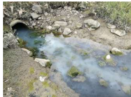
Picture 4: Pipe discharge
