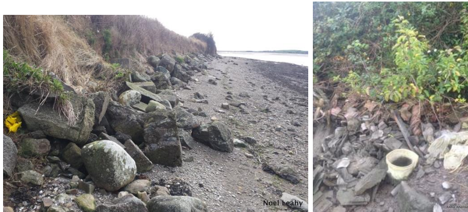
Figure 5. Demolition waste and landfill materials to protect the land against erosion in Bannow Bay and Cork- by Noel Leahy (left) and Anna Aherne (right)
