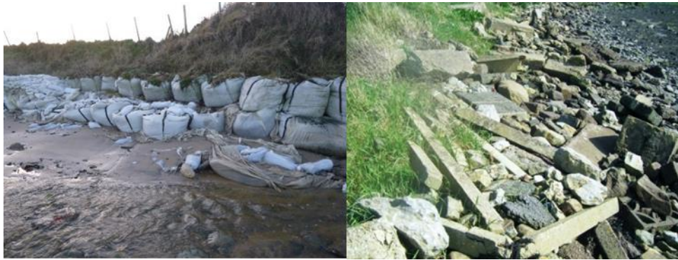
White erosion control sand and mortar sacks which the sea is taking apart at Kilpatrick dunes, Co Wexford (left) and Construction waste dumped onto the edge of the Dungarvan harbour Natura 2000 site is in the same position as in 2012 (right). Picture by surveyor.
