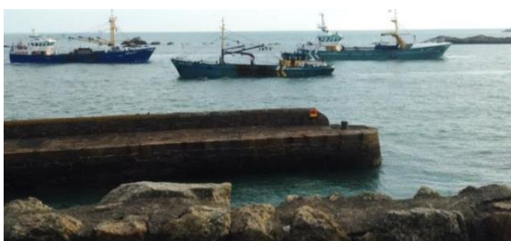
Picture 2. 2 Coliemore harbour. Old sea wall as hard erosion control. Photo Karen Downing
