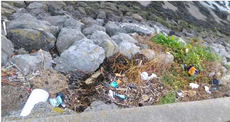
Picture 2. 4 Looking down a rough boulder sea wall, which also acts as marine litter tra.p Photo by Eiméar Manning.
