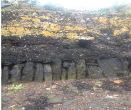
Image 5. "As with other parts of this sea wall in other units that have been surveyed in this general area there is obvious evidence of erosion with the sea wall"- Anna Aherne, Ashgrove. Photo by Anna Aherne
